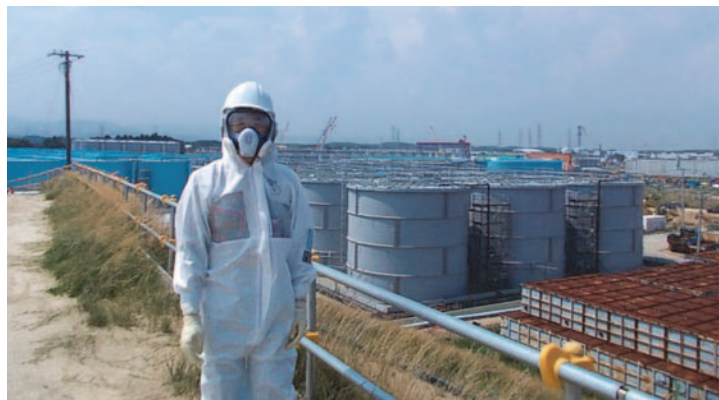
FIGURE 1 Large storage tanks used to house treated contaminated water.
